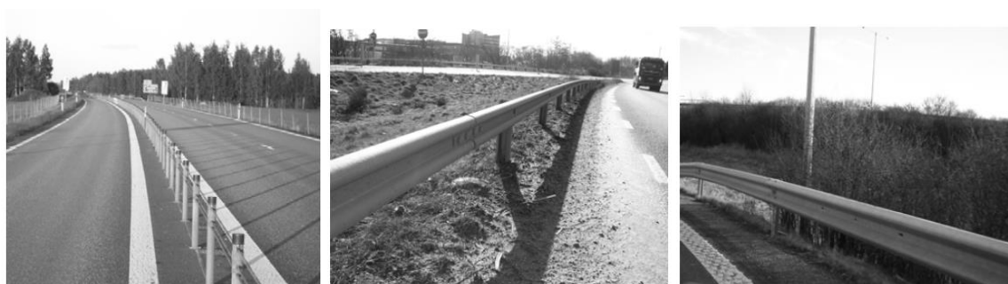
Figure 12: A wire rope barrier (left), a Kohlswa-beam barrier (middle) and a W-beam barrier (right). Source: Karim (2011).
