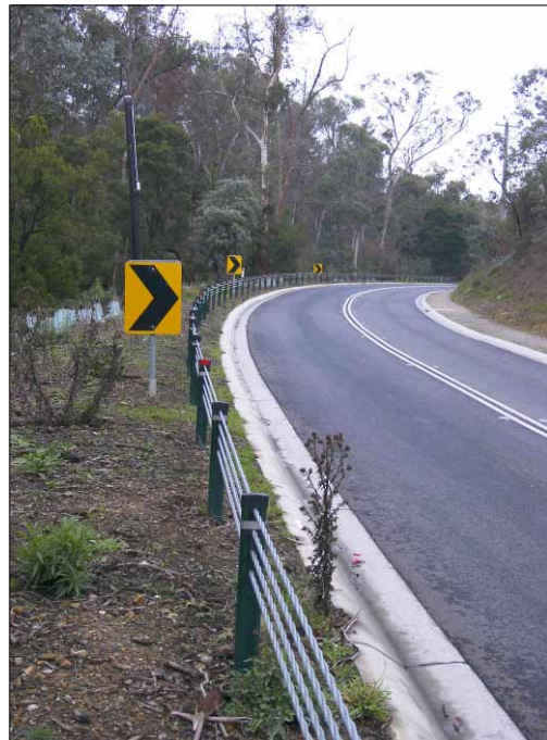
Figure 20 Four rope wire rope barrier
