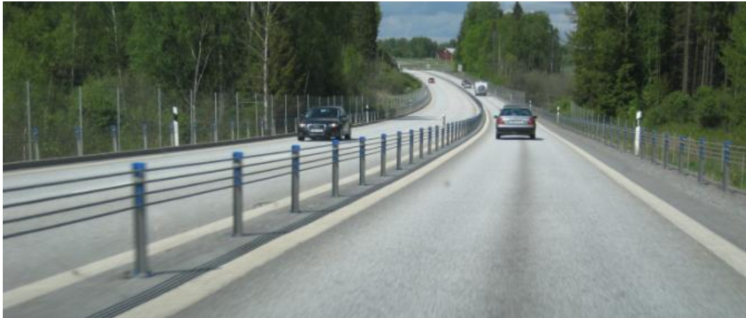
Figure 5: Swedish 2+1 road [source: reproduced with kind permission from Torsten Bergh of a VTI Powerpoint presentation to US AFB 20 Roadside Safety Barrier committee in San Antonio, June 2009]
