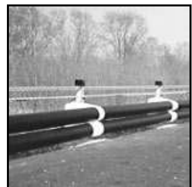
Figure 2 - example of Moto.Tub on site
