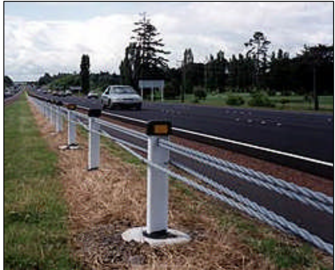
Figure 1: Typical flexible barrier design
