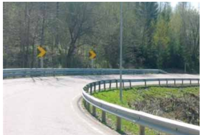
Figure 19. Norwegian Vision Zero Motorcycle Road after brush clearing and installation of motorcycle barrier on outside of curve.
